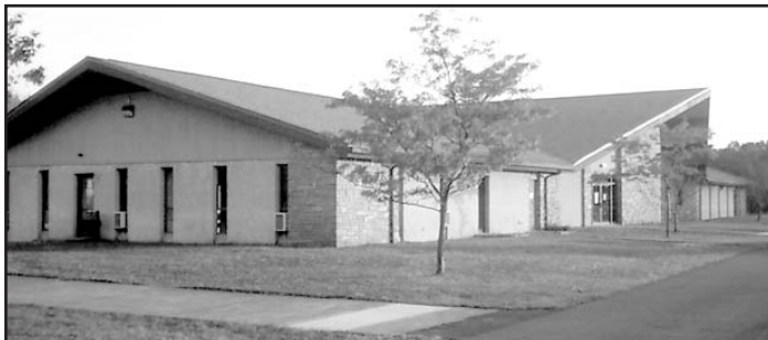
Creative use of a former church enables NCC to better serve students.
